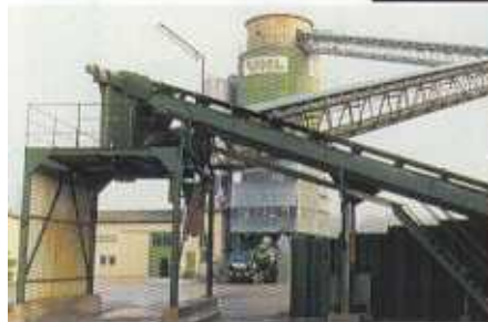
GREASE MAX ® installed at a Quarry
