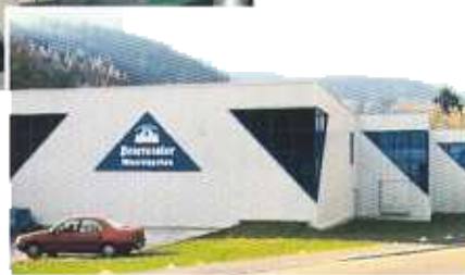
GREASE MAX ® installed at a Mineral water plant
